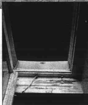
Leaky window – mold is beginning to rot the wooden frame and windowsill.
